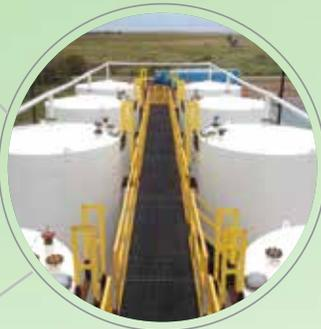
Fibertred® stair treads and Fibergrate moulded grating provide corrosion-resistant walkways and platforms throughout chemical facilities.
