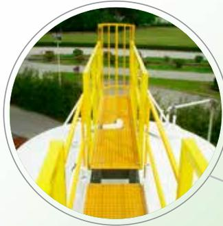
Fibergrate® moulded grating and Dynarail® handrail and ladder systems provide safe access to tanks.
