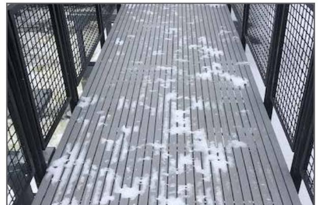
The corrosion resistance of Fibergrate's fiberglass reinforced plastic (FRP) products made this the perfect fit for the wet environment. The walkway will not require constant maintenance and will have a long service life compared to traditional products.
