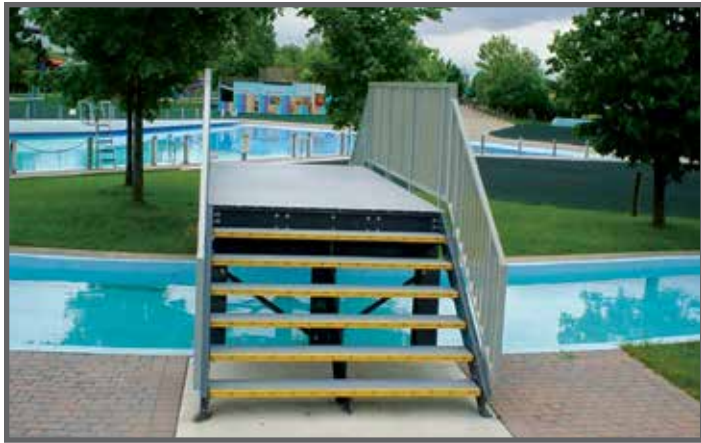
This bridge at a waterpark was constructed using Fibergate's railings, grating, stair treads and structural shapes. In addition to being ADA compliant and slip resistant, this grit-top surface is also barefoot friendly.
